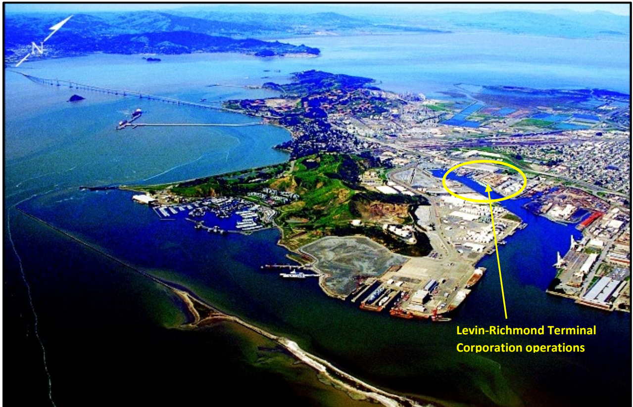
Figure 2 Levin-Richmond Terminal Corporation has operations in the Port of Richmond precinct, located in San Francisco Bay. The port is capable of receiving Panamax sized vessels.
