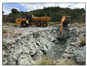
Photo 4: Excavation of Waste Dump
