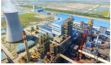
Figure 1 The MOLONG's HIsmelt plant in Shandong Province was the second commercialised plant and achieved its first million tonne of pig iron by December, 2019.
