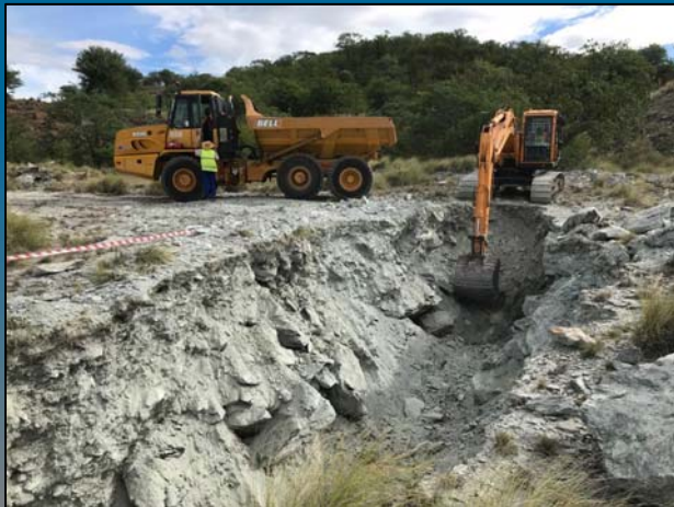
Excavation of waste dump
